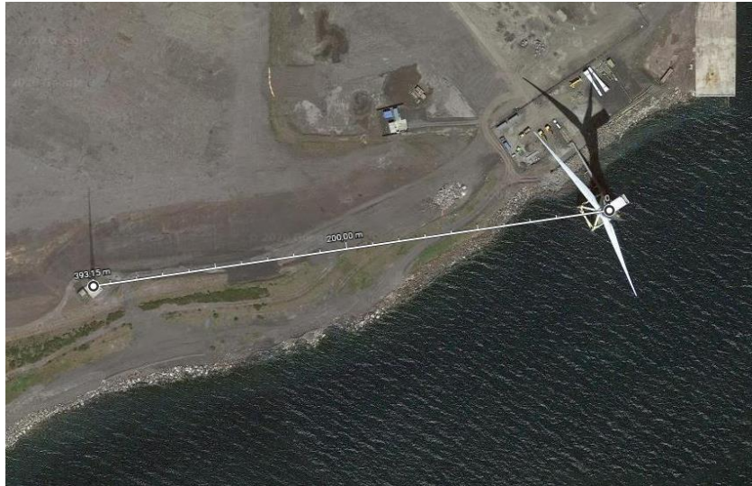
Figure 12 Aerial photo from Google Earth of the LDT and met-mast. The direction between the mast and turbine is 81^\circ
