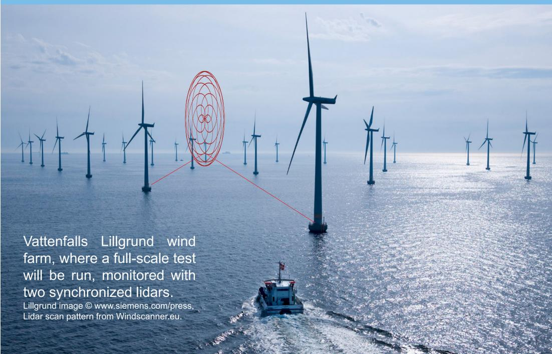
Vattenfalls Lillgrund wind farm, where a full-scale test will be run, monitored with two synchronized lidars.
