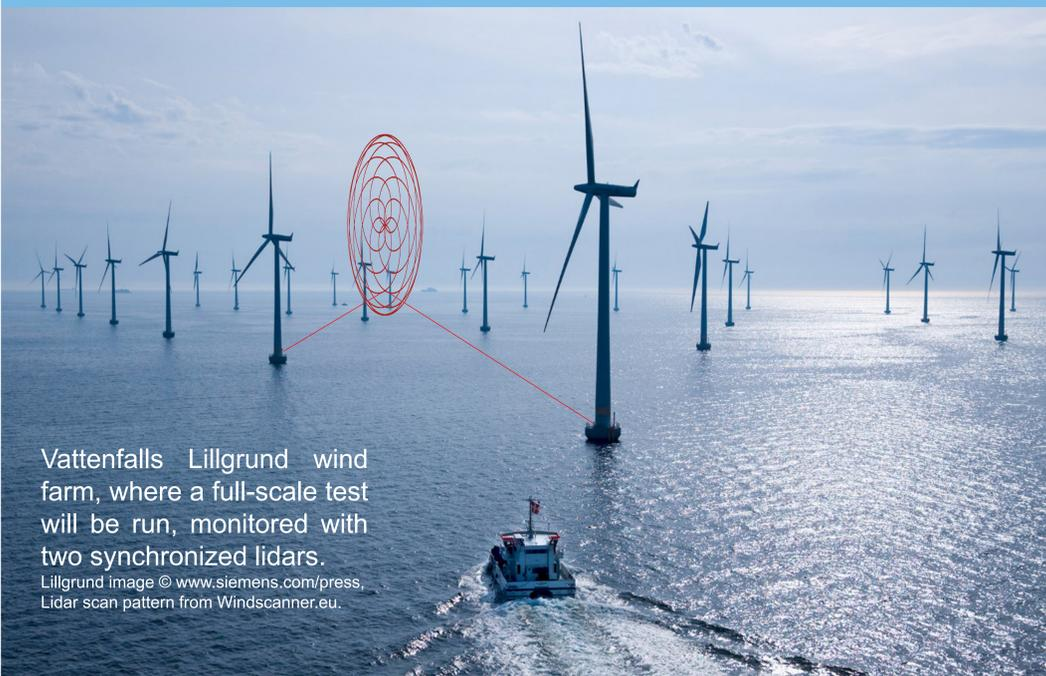
Vattenfalls Lillgrund wind farm, where a full-scale test will be run, monitored with two synchronized lidars. Lillgrund image © www.siemens.com/press. Lidar scan pattern from Windscanner.eu.
