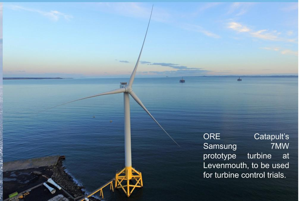
ORE Samsung 7MW prototype turbine at Levenmouth, to be used for turbine control trials.
