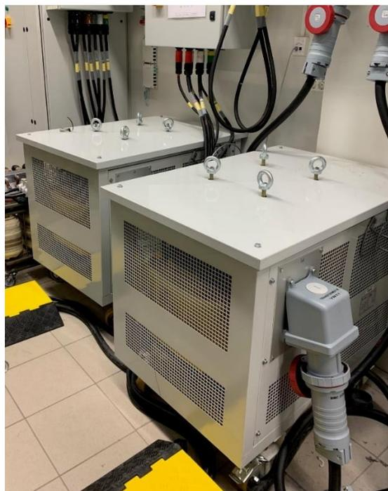
Figure 4-5: Transformers (60 kVA).
