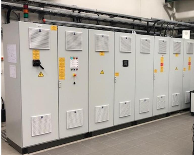
*Figure 4-6: Controlled voltage source (200 kVA).*
